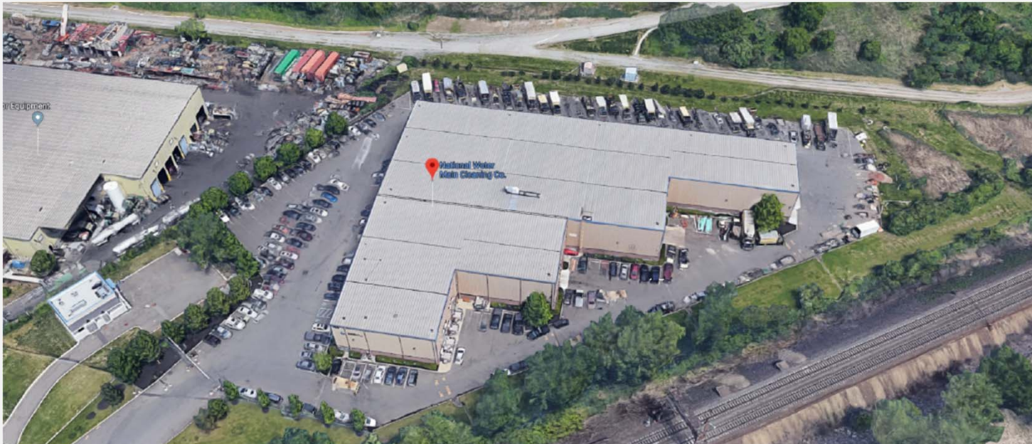
Parcel 113 (1806 Harrison LLC / National Water Main Co.)
